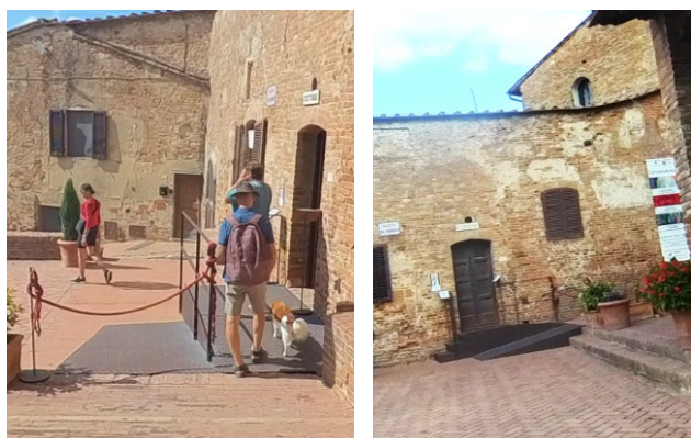
Third entrance ramp
